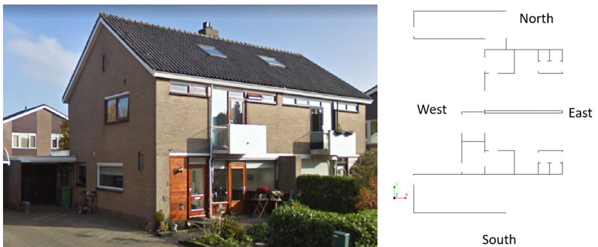
Figure 1. Bleeksteen building semi-detached house. South-East façade view (left) and plan view (right).
