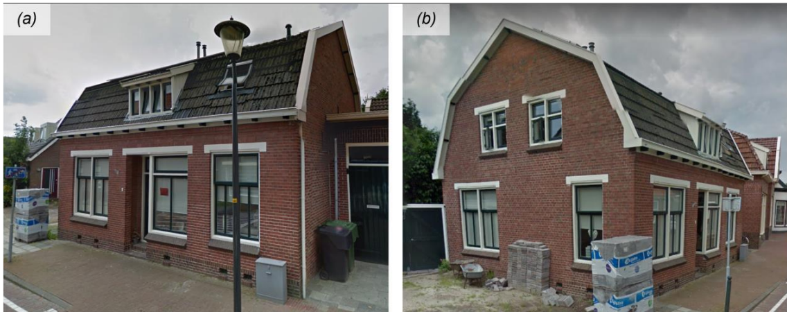
Figure 4: Building views, a) North-East view, b) South-East view (from [4]).
